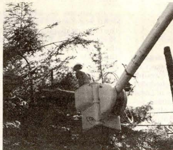
Working Foreman Walt Vance trims limbs from power line obstruction.
