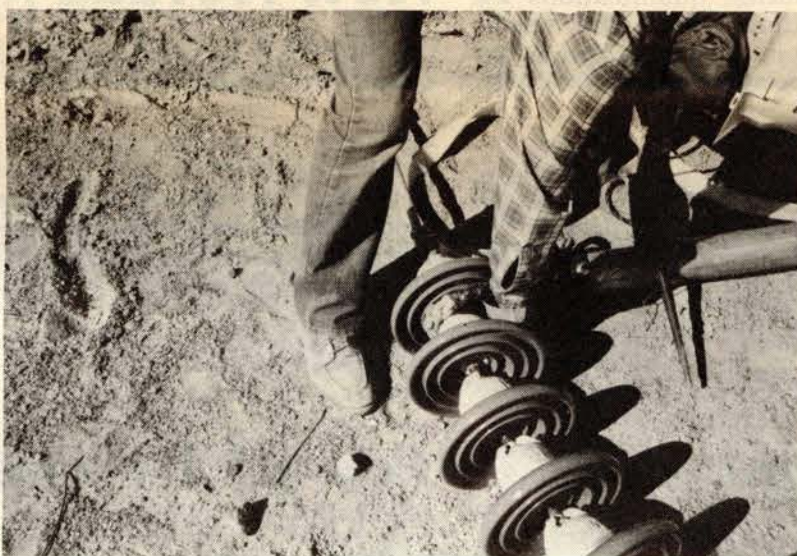
Lineman rigging insulators for insulation by helicopter.
