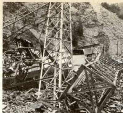
Downed switchyard towers and crushed electrical apparatus.
