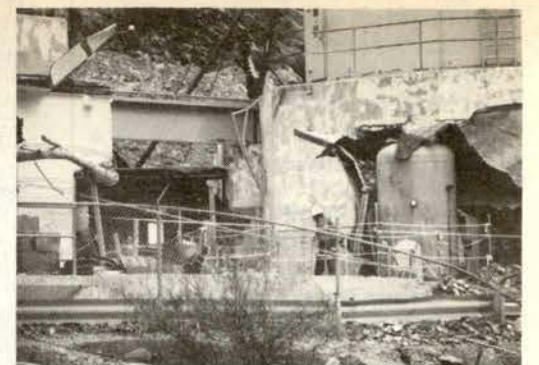
Severely damaged unmanned Caribou #2 Power House, right.
