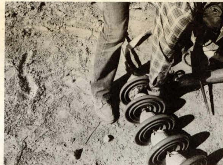
Lineman rigging insulators for insulation by helicopter.
