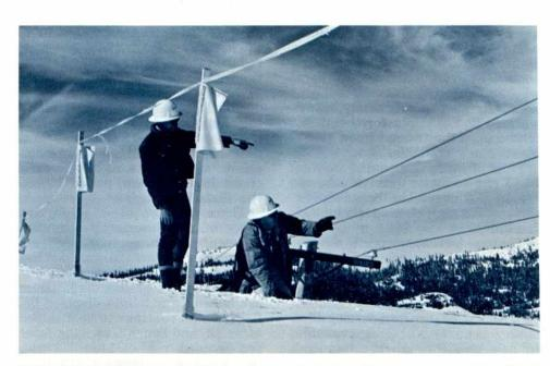
DANGER ZONE — Bright colored flags and high voltage signs warning skiers of danger have been installed by Pacific Gas and Electric Company crews along nearly buried power lines on some Sierra ridges. These PG&E men were members of a crew which installed a 25-foot extension on this 45-foot pole near Boreal Ridge in Nevada County to raise the power line higher.
