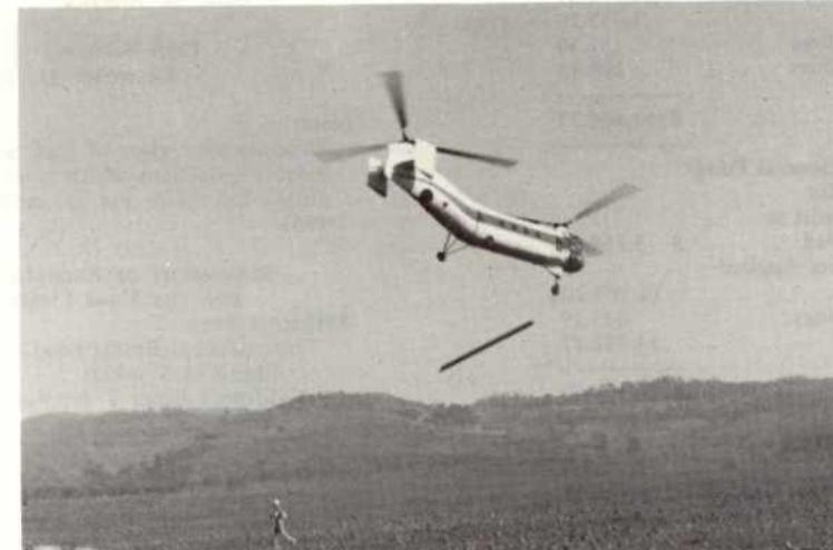
3. Loaded with a bundle of steel, the 'copter takes off and heads northeast to a distant tower site, such as Dry Creek, on the Pacific Northwest-Southwest Intertie.
