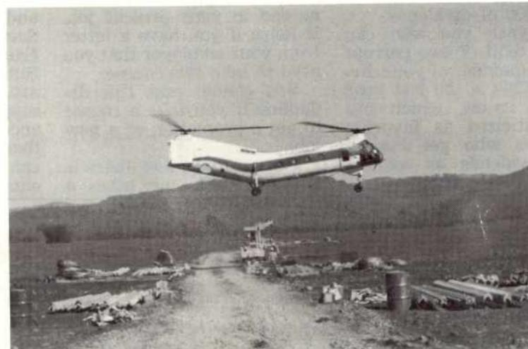
2. The helicopter hovers over tower steel brought out from the Chico G.C. yard, while men on the ground guide the pick up.
